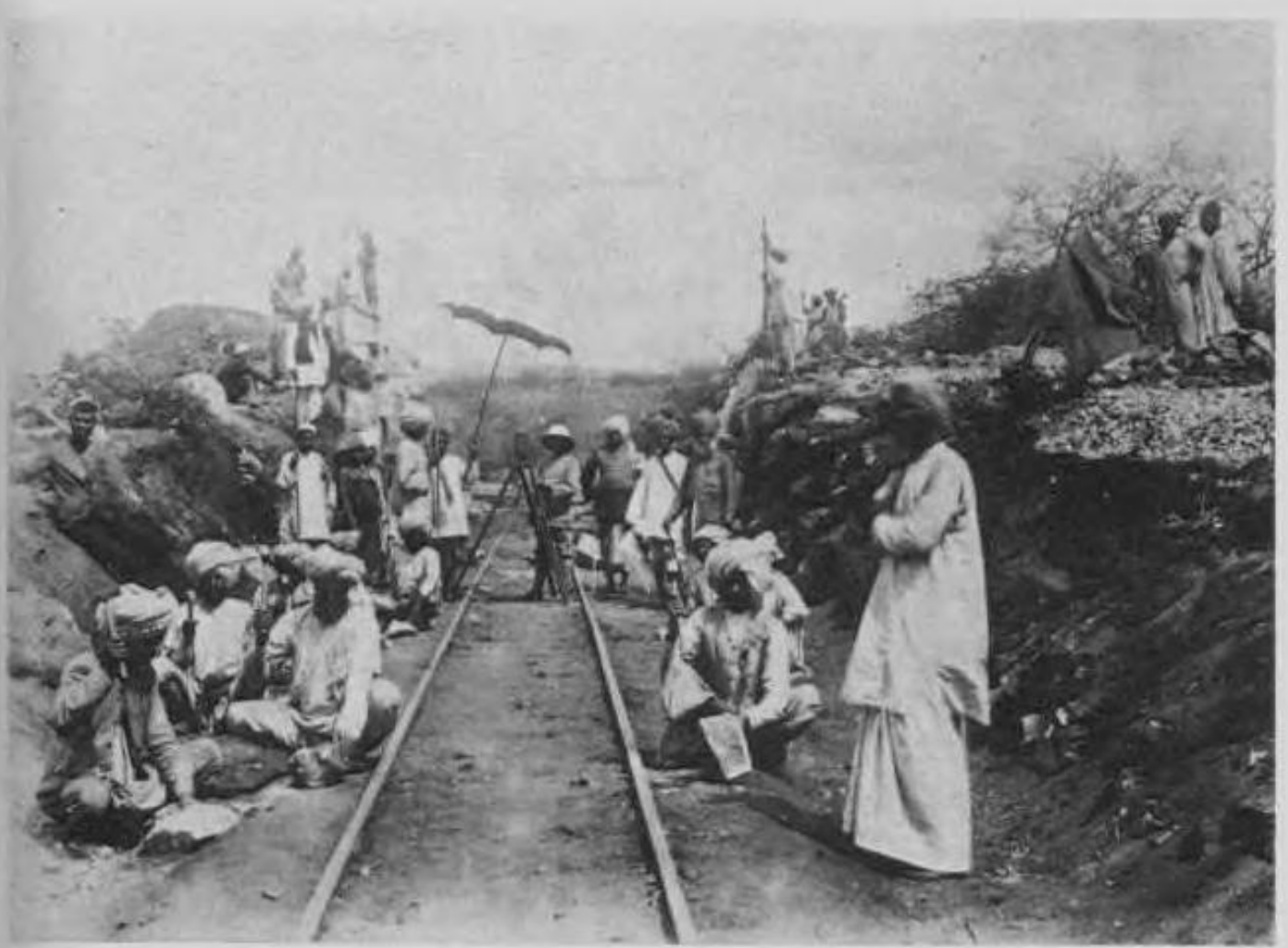
20 Railway builders: Indian coolies laying the track
