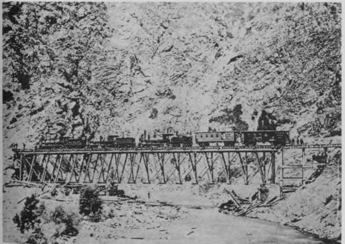
21 Devil's Gate Bridge during the construction of the Union Pacific Railroad
