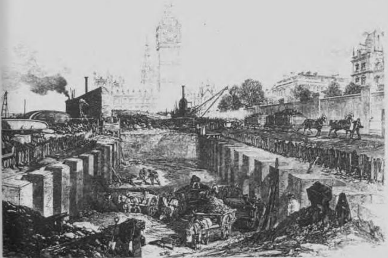
5 Shovel, barrow, cart and crane: building the underground railway, London 1869
